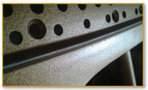
A force of from 16 to 18 tons is applied to a plate when it is strung and tuned. The plate must have sufficient structural strength to withstand this pressure and deliver acoustical response as well. Kayserburg Artist Series pianos have plates which are designed by craftsmen whose engineering excellence incorporates, in each plate, the ability to achieve maximum tolerances while delivering distinct acoustical responses. Each Kayserburg receives a plate which has
